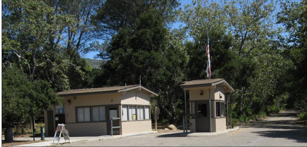
Figure 2-4. Current entrance kiosk and office.
