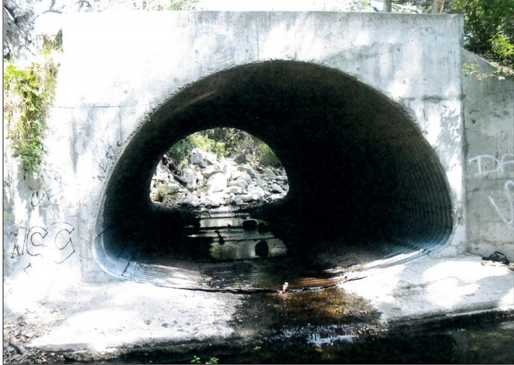
Figure 2-6. Close up of culvert at El Capitán Creek crossing.
